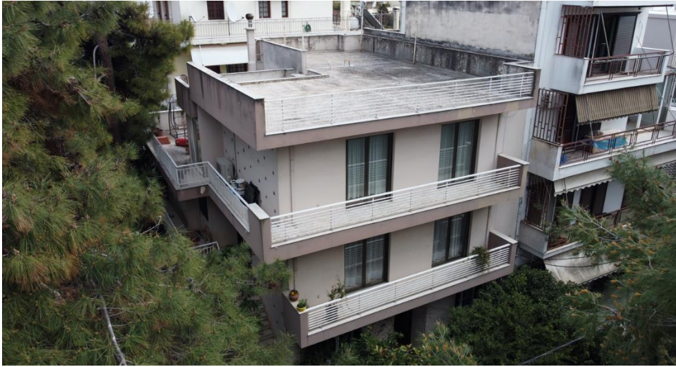
CS4 as seen from a neighbouring building, before refurbishment
