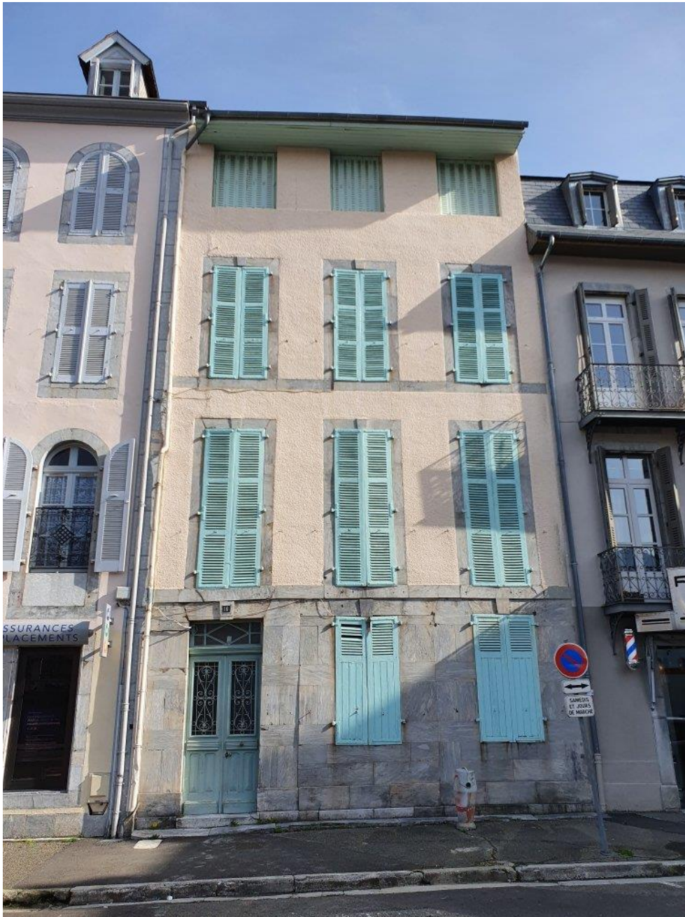
CS7 as seen from the street before refurbishment
