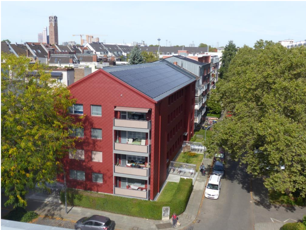
OP39 as seen from a neighbouring building from ca. 165° (south-east)
