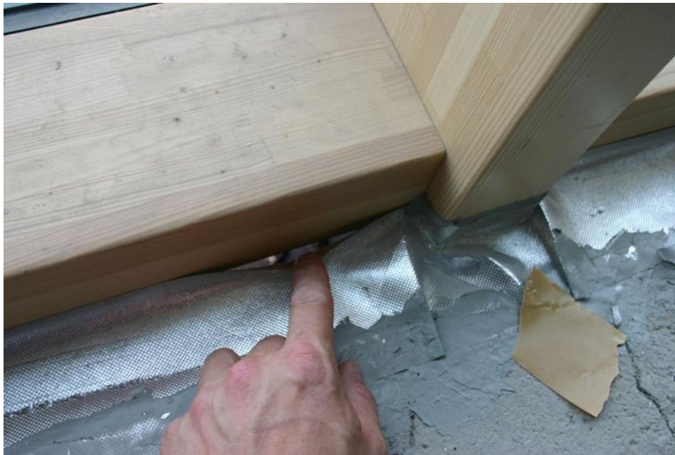
Figure 33: Window installation in a passive house.
