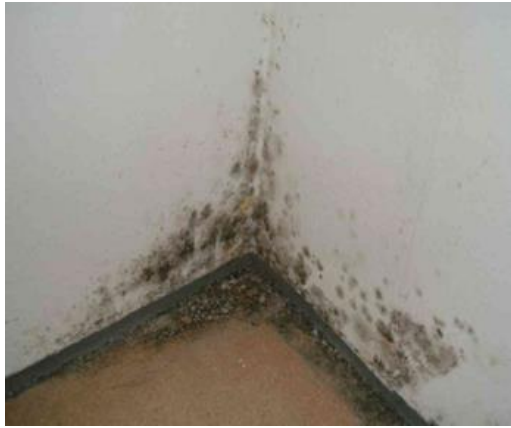
Figure 26: Retrofitting without taking into consideration the thermal bridges.
